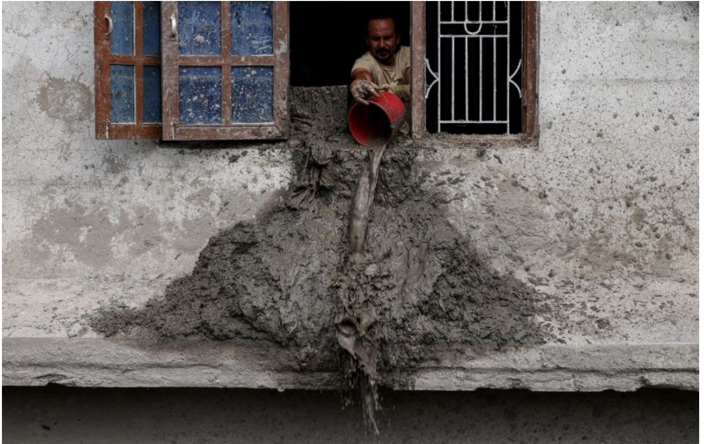
A man pours mud out of a window of a flood-damaged home following deadly flash floods and a mudslide, in Devighat, Nuwakot district, Nepal, September 10. REUTERS/Tyrone Siu
